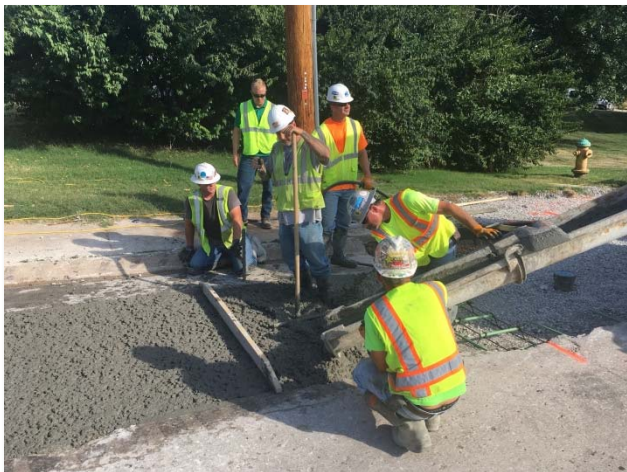
Union Road concrete pavement repair
